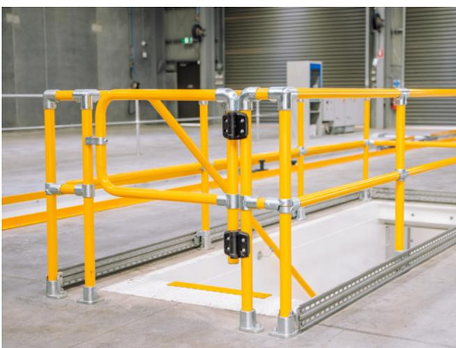
“On platforms and landings, guardrails are required when it is not safe to step or stand outside the walkway without risk of falling.”
