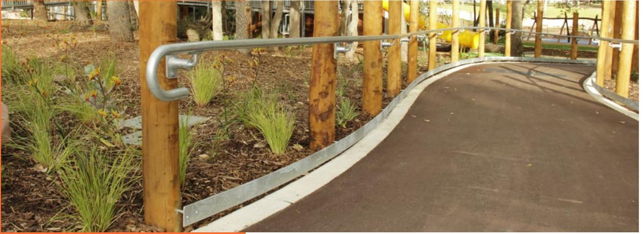
A kerbrail system is required on ramps and their intermediate landings;
